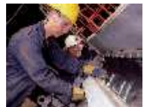
Expansion joint installation
