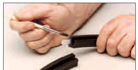
**Stage 1:** Apply epoxy adhesive to joint faces of Walkersele® OSJ.
